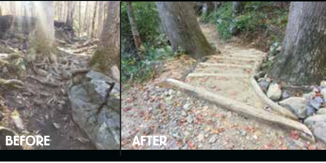
BEFORE - Along the Rainbow Falls Trail, an example of trail trenching with exposed roots and no drainage, before the problems were addressed by the Trails Forever crew.
